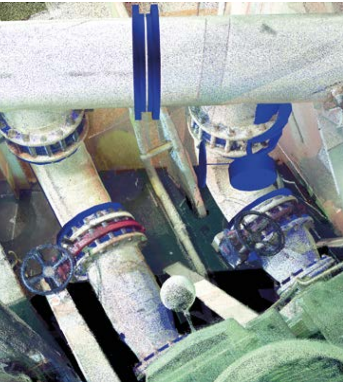
Rubber-lined seawater cooling...
